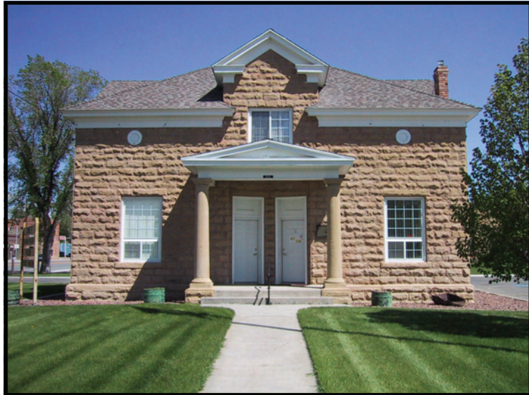
Cowley's historic town office building
